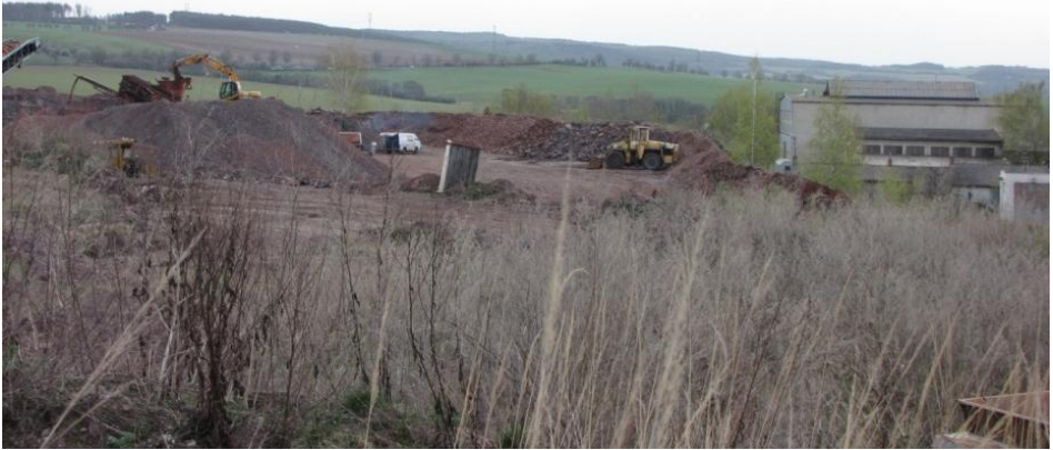
Fig. 3: Waste rock removing from the former Kukla Mine area
