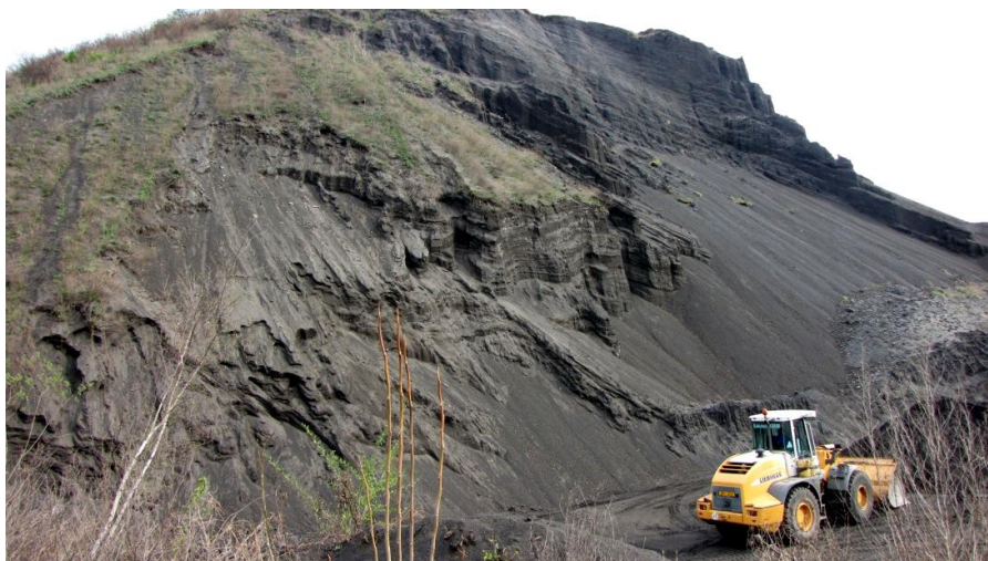
Fig. 5: Coal ash removal by Prefa company
