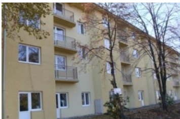
Picture 3: Construction of New Housing Units in the Village of Jarok
