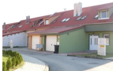
Picture 4: Construction of Two-house Units in the Village of Branč
