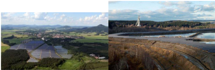
Fig. 3: Solar power station Ralsko Ra 1 in former military area and solar power station Rožná (DIAMO I.) in the area of uranium mining.
