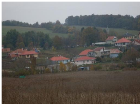
Picture 1: Individual Construction of Family Houses in the Village of Golianovo
