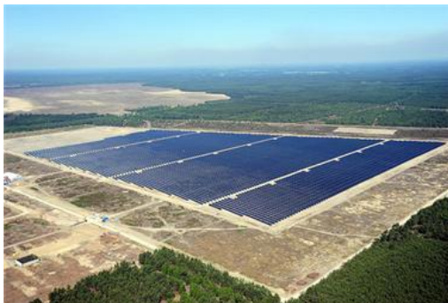
Fig. 2: Photovoltaic power station Lieberose in Germany
